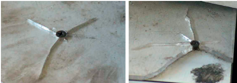
Figure 3.44 Catastrophic failure with use of flat head screw in acrylic sheet
