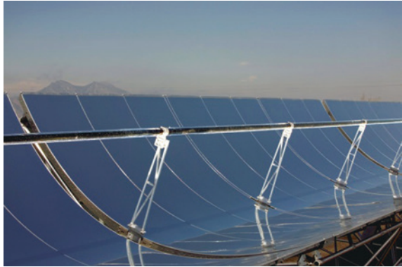
Fig. 2.4 Parabolic trough concentrating solar collectors with heat transfer fluid in the tubing absorbing thermal energy ( http://energy.gov/eere/renewables/solar )
