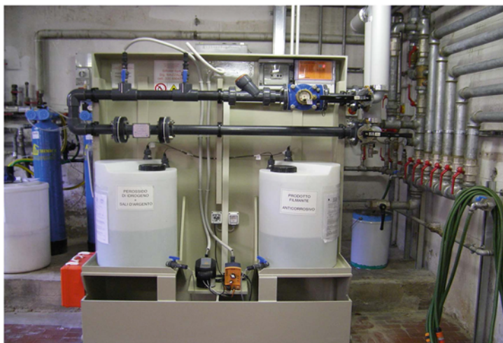
Fig. 2.2 Water decontamination in food plants has to be considered as one of the main pilasters of food safety. The complete purification or production of potable water is not possible in several food production environments. For this reason, food business operators can reasonably use only a few selected methods for decontaminating water supplies from the microbiological viewpoint. One of these strategies is the use of innovative systems such as hydrogen peroxide and silver ion generators
