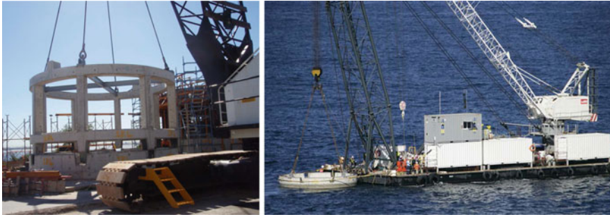
Fig. 2.14 Pre-cast intake coarse screen structure/screen base being lowered
