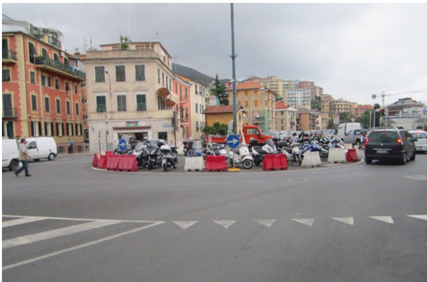
Fig. 2.11 Assembly roundabout with motorbikes' parking at central island; near Italian border with France
