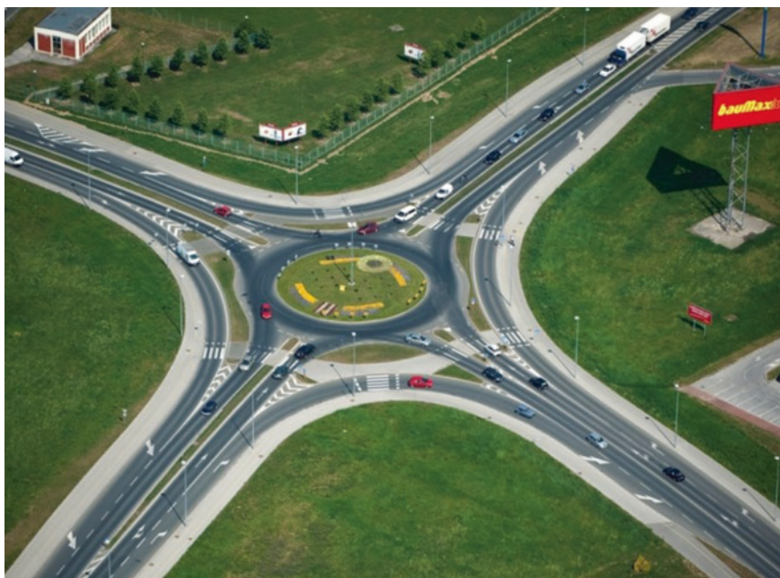
Fig. 2.54 Roundabout with four segregated right-hand turning acceleration lanes; City of Varaždin, Croatia
