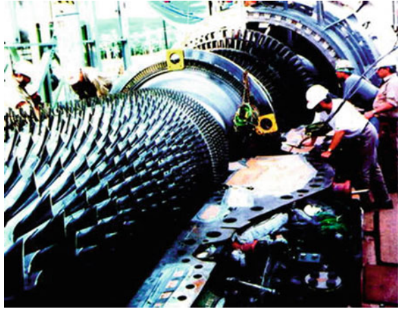
Fig. 2.4 Inspection of a steam turbine
