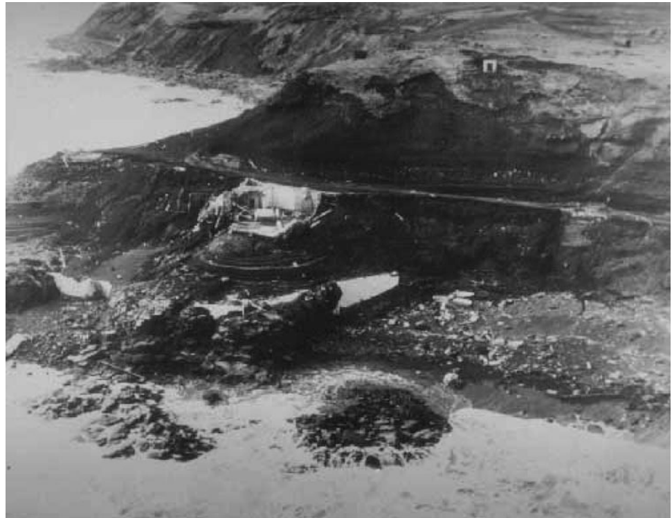
Fig. 2.8 The remains of the Scotch Cap lighthouse, Unimak island, Alaska, following the April 1, 1946 Tsunami. A coast guard station, situated at the top of the cliff 32 m above sea level, was also destroyed. Five men in the lighthouse at the time perished. Source United States Department of Commerce, National Geophysical Data Center
