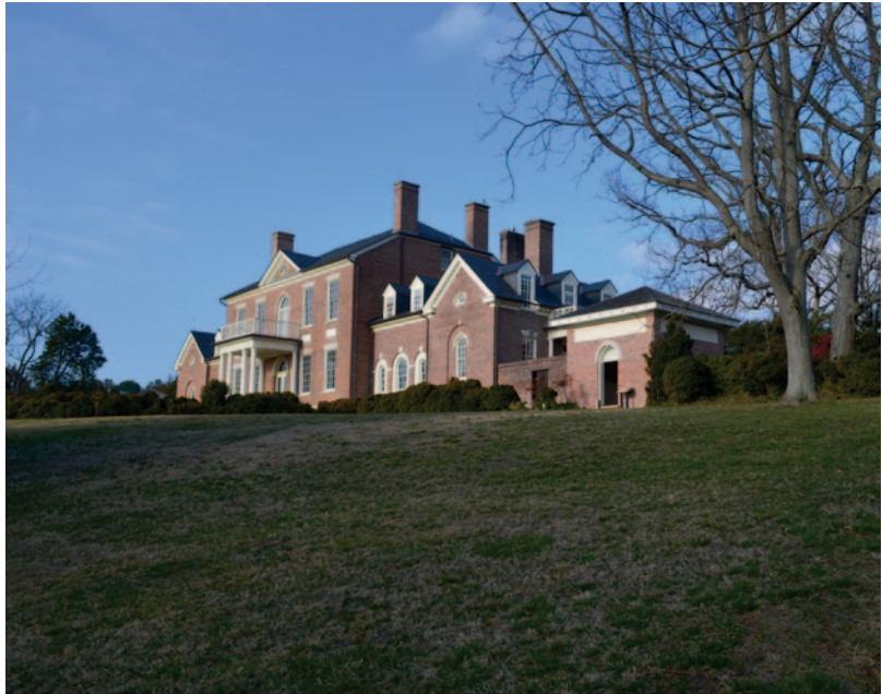
Fig. 2.2 “Woodlawn,” another historic estate, was to be sold to Belgian monks until the Historic Woodlawn Public Foundation stepped in to save it, transferring it to the National Trust as the organization’s first house museum. (Author’s photograph)
