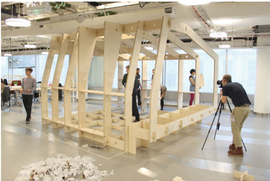
Fig. 2.12 WikiHouse plywood skeleton (© WikiHouse)
