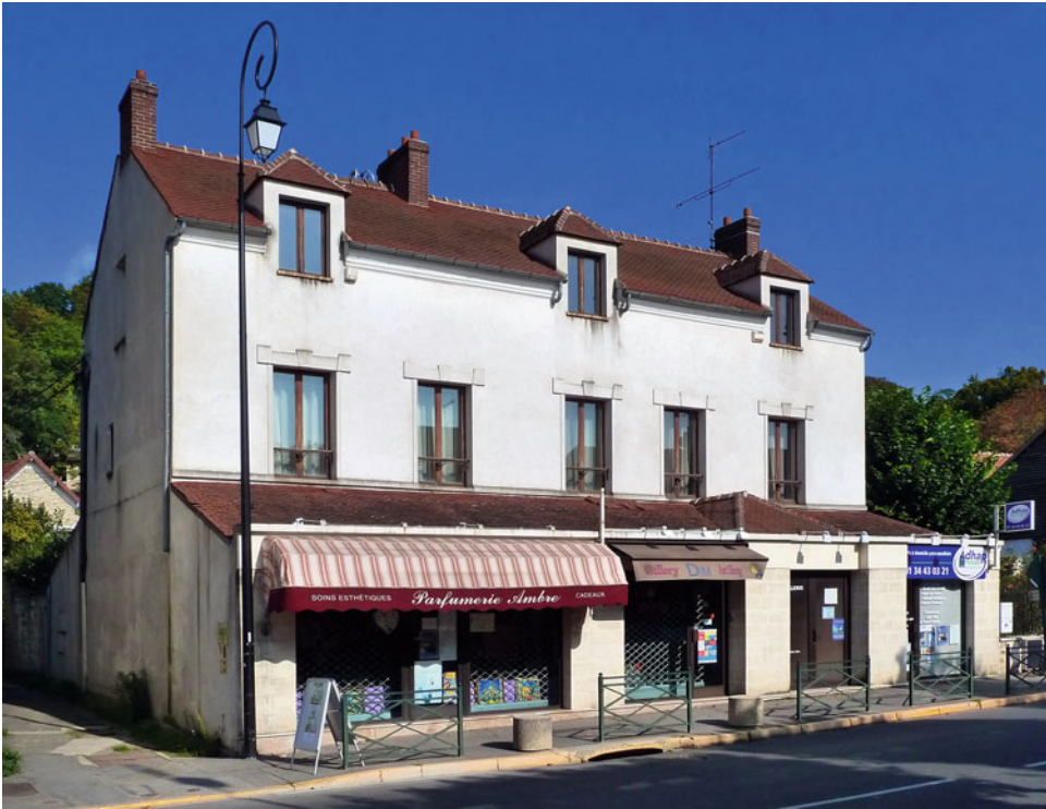
Fig. 2.5 Several guidebooks incorrectly direct visitors to this house at number 44 Rue du Général de Gaulle. The sunlight illuminates the south-facing facade in this midday photograph, but in spring and summer the Sun's rays do not illuminate the front of the house near sunrise or sunset (Photograph by the author)
