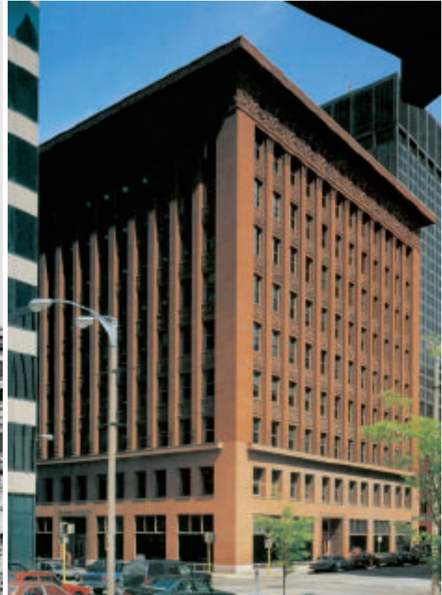
Louis Sullivan, Dankmar Adler, Wainwright Building, St. Louis, 1890–91
