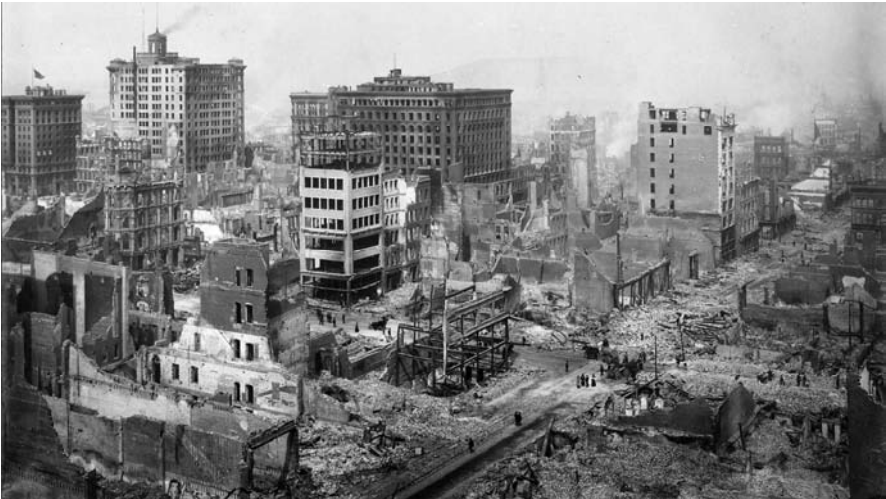
Fig. 1.3. Earthquake damage in San Francisco after the 1906 earthquake.
