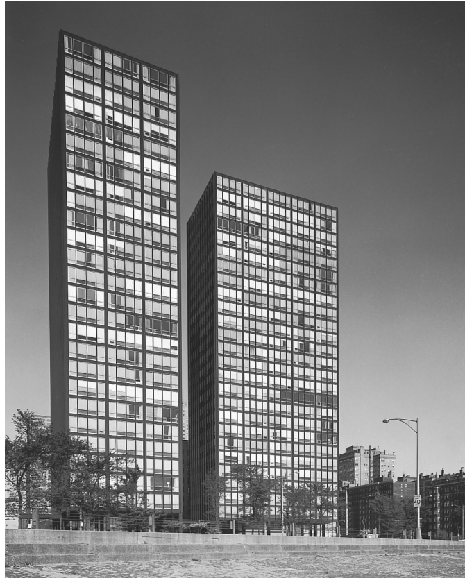
Figure 1.6. Mies van der Rohe, 860–880 Lake Shore Drive (1949–51). (Credit: Ezra Stoller © Esto.)
