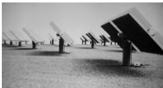
Fig. 1.4. The 350-kWp SOLERAS project power plant was the world’s first and largest concentration plant. It was built and deployed in Saudi Arabia, using the evolution of Sandia Labs (technology by Martin Marietta)
