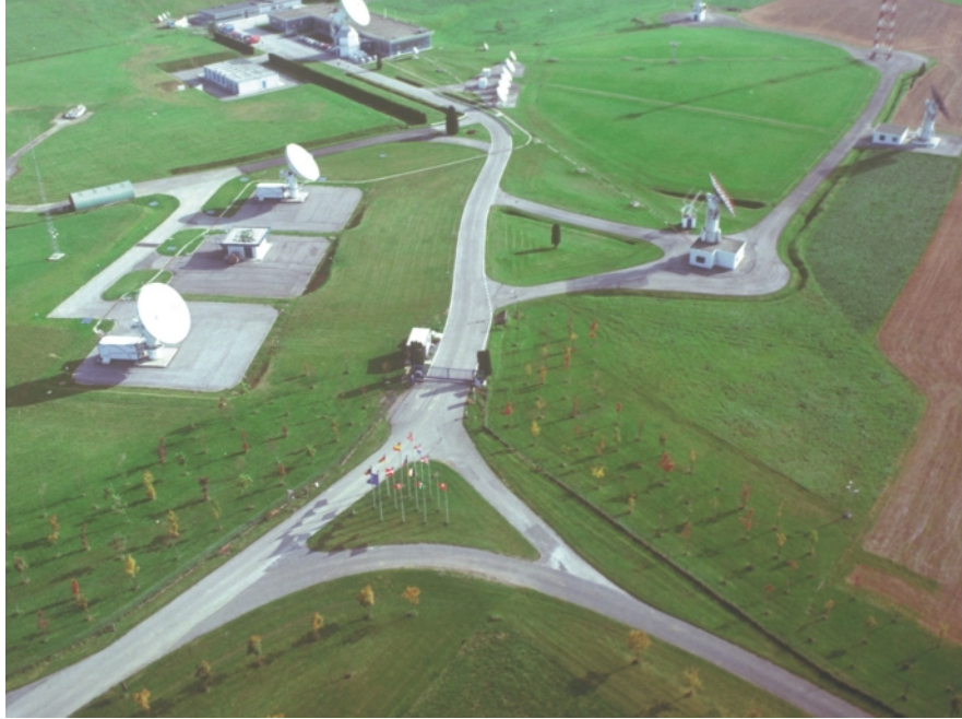
Fig. 1.8. The ground station complex at Redu, Belgium, provides telemetry, tracking, and telecommand operations for low-Earth and geostationary satellites (courtesy ESA)
